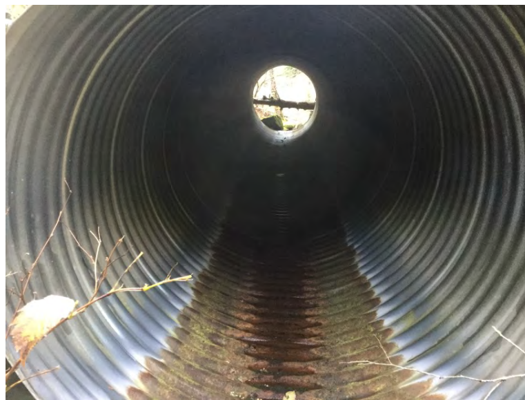
Looking through culvert from inlet
